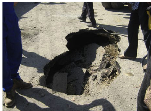
(b) Street subsidence
